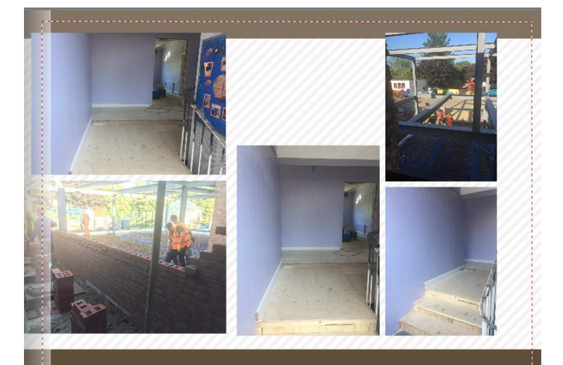
At the end of the summer the extension had lower floor external walls and the path to the emergency exit to the school had been repaired and re-laid. Internal walls had been demolished and rebuilt to create a large upper floor classroom and two storage rooms. All walls had been re-plastered and painted. New toilets had been installed and a remodelled staircase and lobby area had been created.
